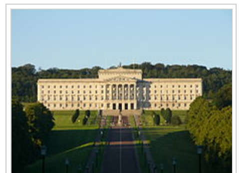
Parliament Buildings at Stormont, Belfast, seat of the assembly.
