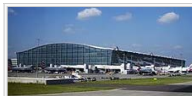
Heathrow Terminal 5 building . London Heathrow Airport handles the most international passenger traffic of any airport in the world. [125][126]
